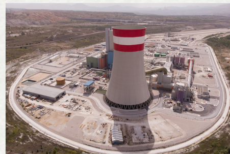
PTOLEMAIDA 5, THE LAST NEW COAL PLANT IN GREECE
